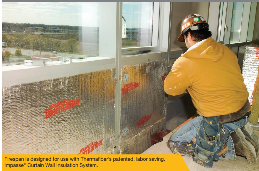
Thermafiber insulation provides the critical components of the perimeter fire containment system in the Trump International Hotel and Tower in Chicago.
